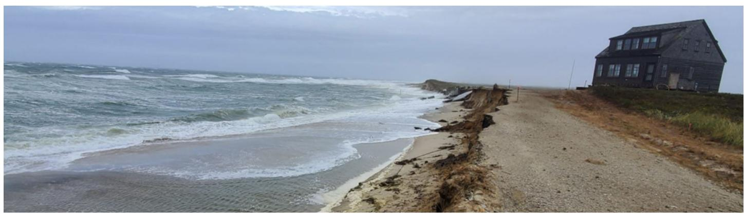
Figure 21. Coastal erosion impacting a private access road, September 2020
