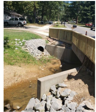
Box culvert with sidewalk.
