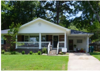
A single-family home with carport.
