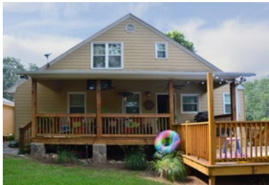
A deck attached to the principal structure.
