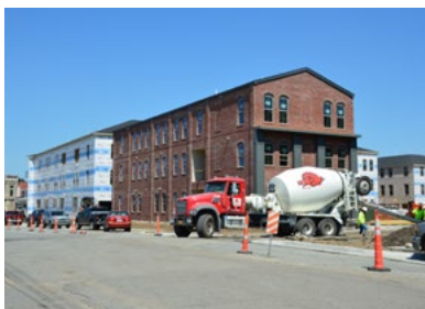
The two buildings pictured above would require site plan review.
