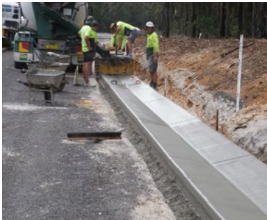
Concrete Valley. Photo: https://www.seattlewapaving.com/concrete-paving.html
