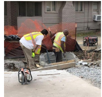
Drainage improvements under construction.
