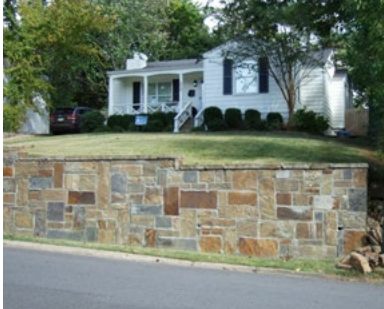
A retaining wall.
