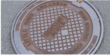
A sewer manhole cover.
