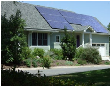
Roof mounted solar panels.
