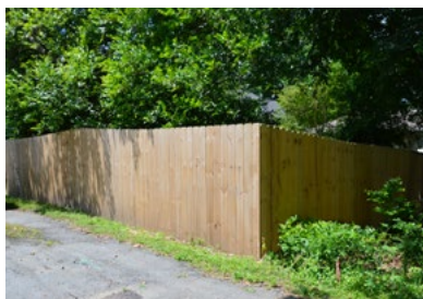
A side yard fence.
