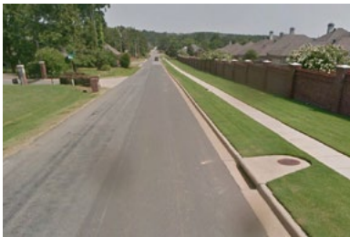
The developer of the subdivision on the right has installed half-street improvements on the boundary street per the Master Street Plan and Subdivision standards.
