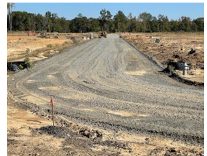
A new street under construction.
