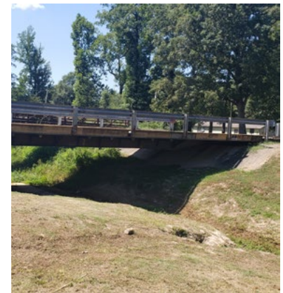
Bridge over a drainage path.
