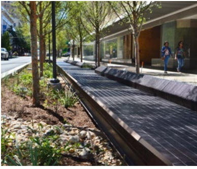
Green Infrastructure like that pictured above uses or mimics natural processes that result in the infiltration and/or evapotranspiration of stormwater in ways that protect water quality. For more guidance on Green Infrastructure for roads, alleys, and parking lots, visit www.epa.gov/nps/green-streets-handbook .
