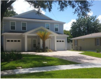
This duplex features a narrow driveway opening at the sidewalk, which then widens to accommodate two garages and additional parking. Image: Bungalower
