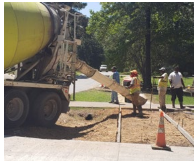
A sidewalk under construction.
