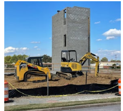
A commercial building under construction.
