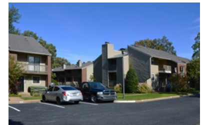
Single-family attached units.
