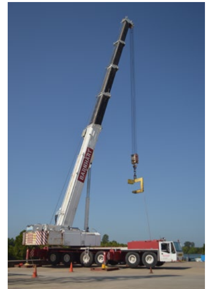
The industrial zone provides space for heavy equipment and operations.
