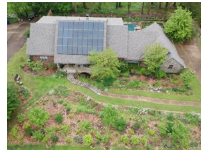
Roof-mounted solar panels. Photo: Layet Johnson
