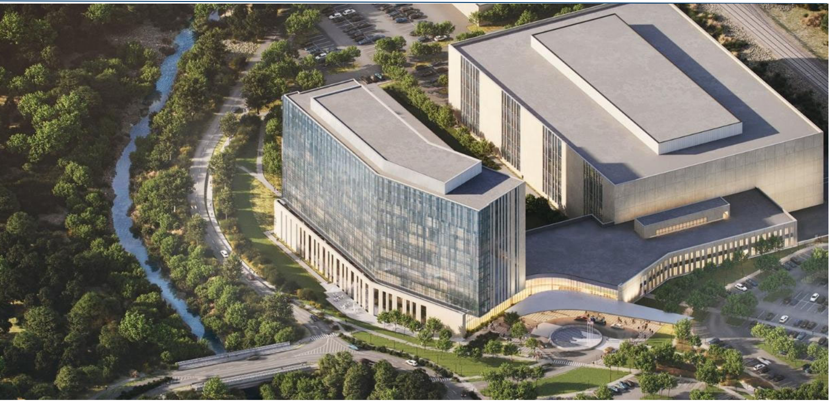
City of Indianapolis
