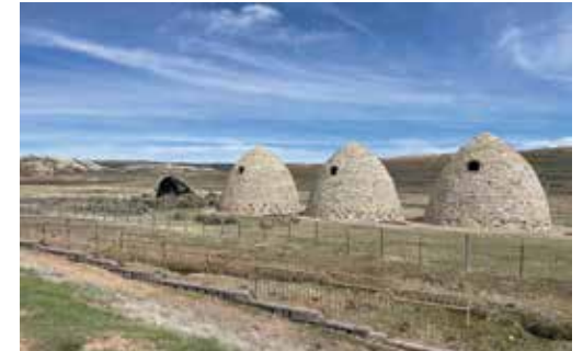
Laima Swanson - Conical-Shaped Charcoal Kilns Built from Local Sandstone and Limestone. Built around 1869 by Moses Byrne near the Union Pacific Railroad in southwestern Wyoming.
