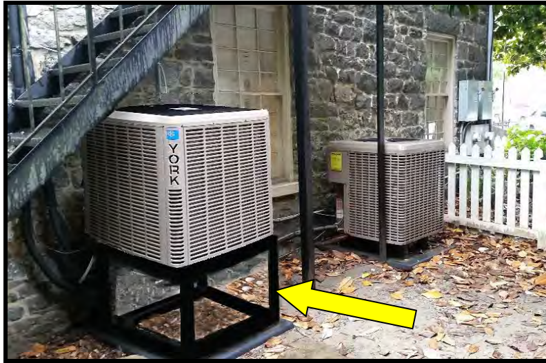
FIGURE 5.14: EXAMPLE OF ELEVATION OF UTILITIES
