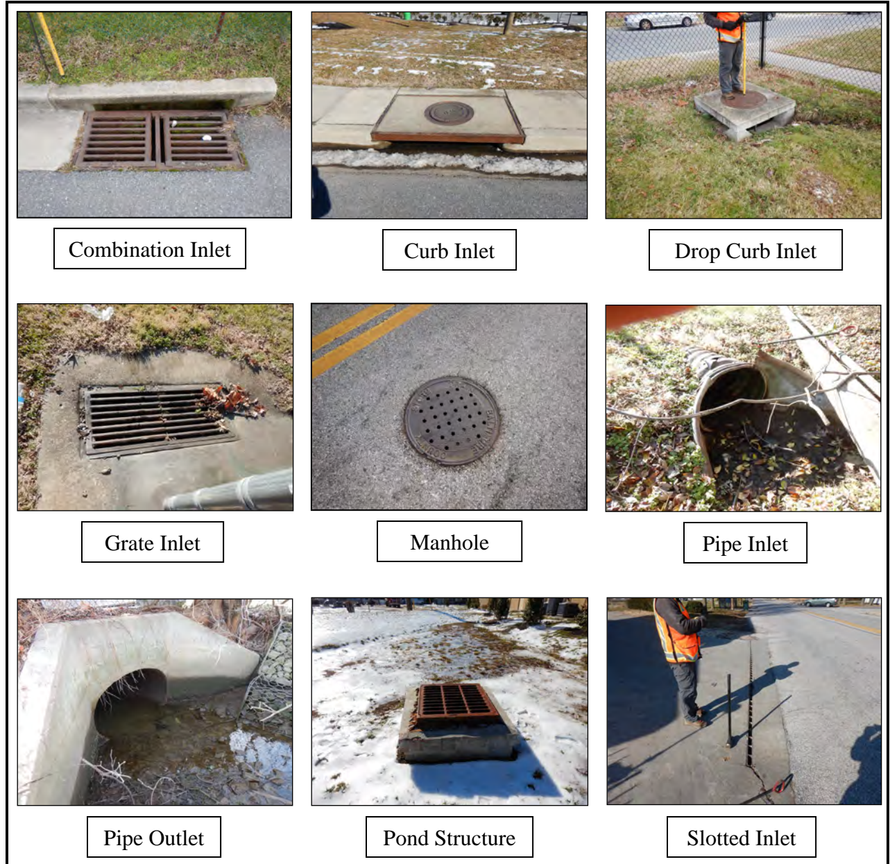
FIGURE 2.1: TYPES OF STORMWATER STRUCTURES IN TURNER STATION
