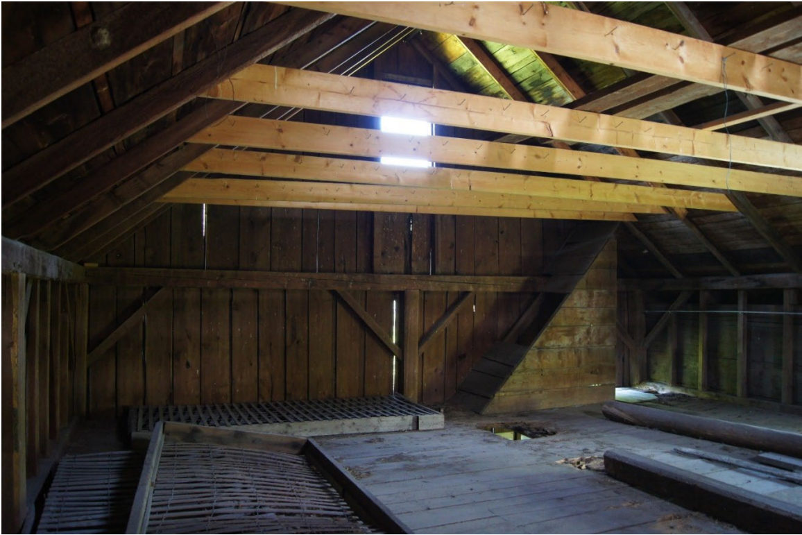
Photograph 56: 5 Home Farm Way, hay loft over barn, note mixture of original framing and cross bracing.
