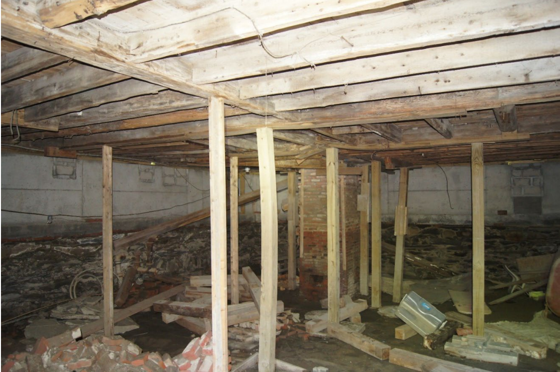
Photograph 58: 5 Home Farm Way, partial basement, note built-up concrete perimeter foundation.
