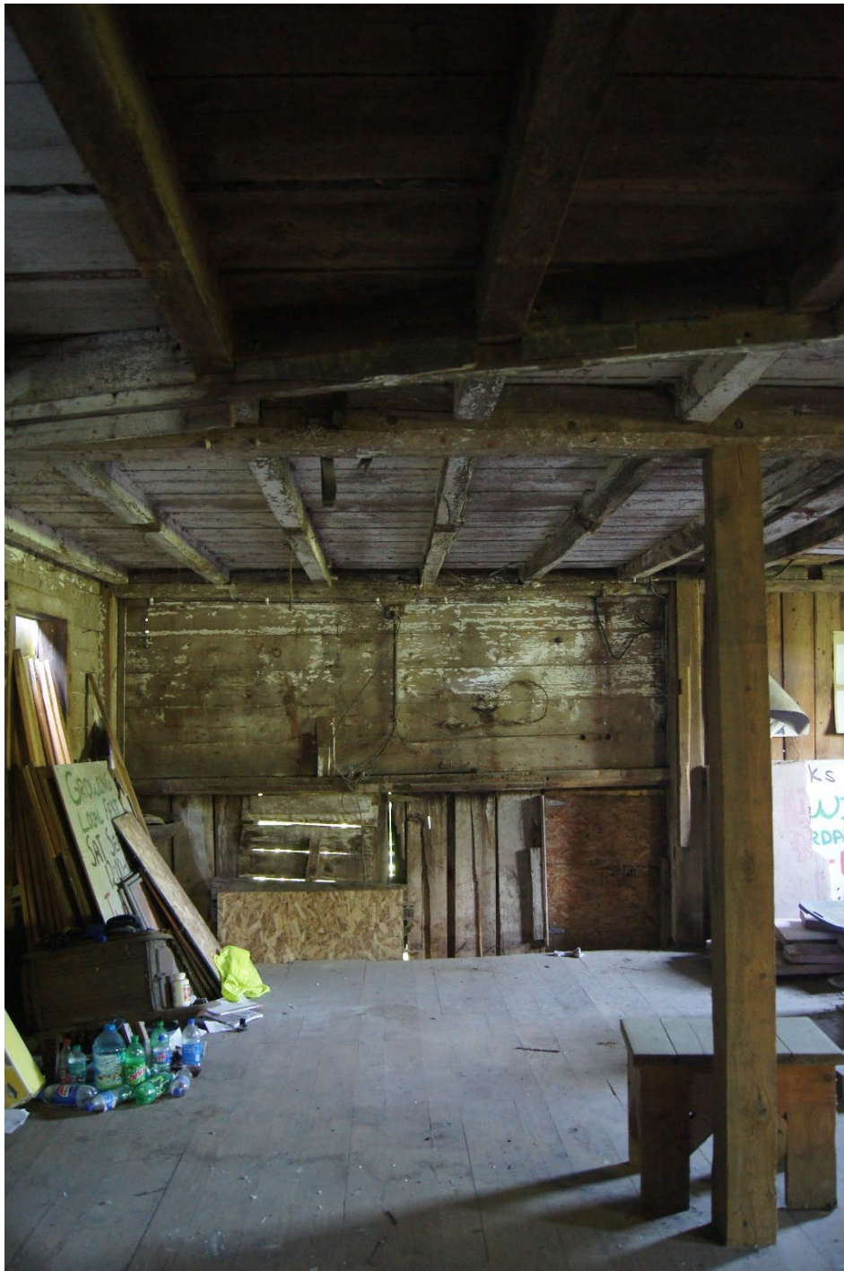
Photograph 37: 5 Home Farm Way, looking west through barn. Hinged opening on wall correlated with horse stalls, since removed.
