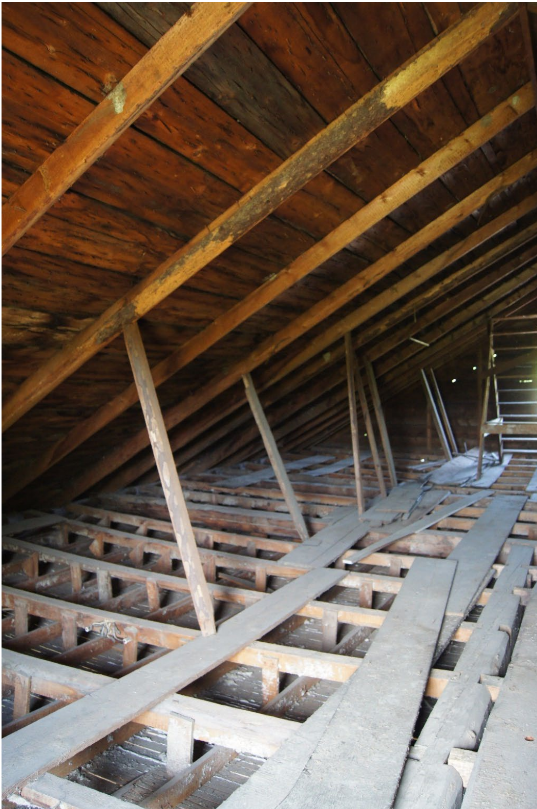
Photograph 53: 5 Home Farm Way, attic detail with built up framing over plaster and lath ceiling.
