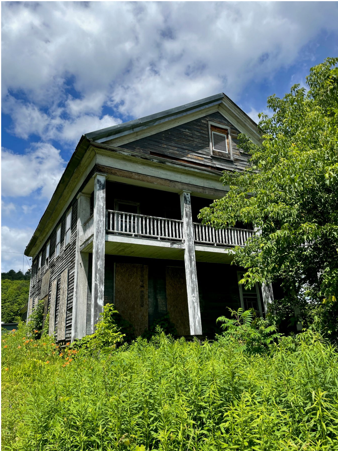
Photograph 11: Detail of 5 Home Farm Way portico, note missing first level porch, removed when building was raised, facing northwest. Photograph Preservation Trust of Vermont 2022.
