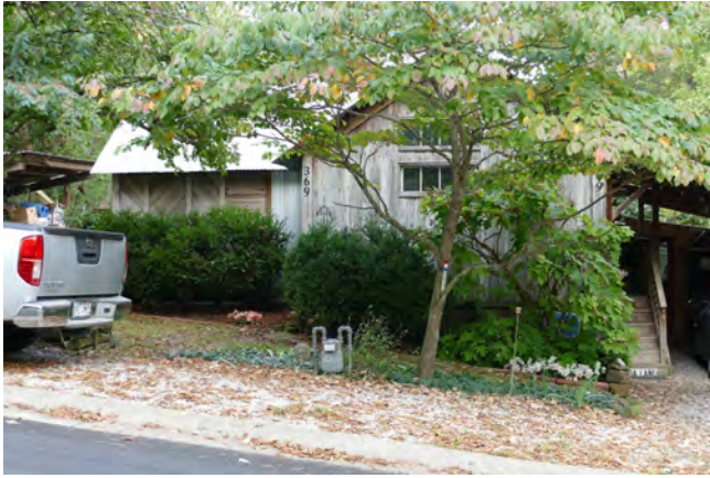
369 E. Center Street Approximate date of construction: 1889 (CAD) Form/Style: Gabled Ell Notes: Extent of alterations unclear
