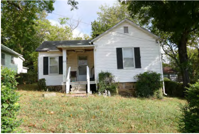
212 E. Center Street Approximate date of construction: 1930 (CAD) Form/Style: Gabled Ell/ "Bent House"
