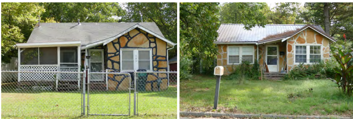
Figure 50 (left): 506 S. Willow Ave features a Giraffe Rock exterior with black mortar. Figure 51 (right): 440 S. Willow Ave features Giraffe Rock with light colored mortar. Both houses were constructed ca. 1930. Post Oak photos 2024.
