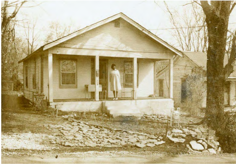
Figure 36. 1972 photograph of 154 E. Meadow Street (extant as of 2024, though damaged by recent fire). Taken by the City Code Compliance department, the house was filed under “structures brought up to standard.” Source: City of Fayetteville.
