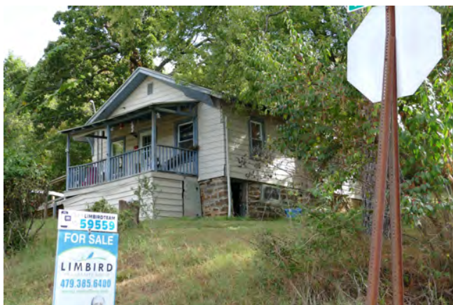
234 S. Willow Ave Approximate date of construction: 1905 (CAD) Form/Style: Gable Front
