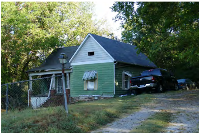
410 E. Center Street Approximate date of construction: 1925 (CAD) Form/Style: Gabled Ell/ "Bent House"
