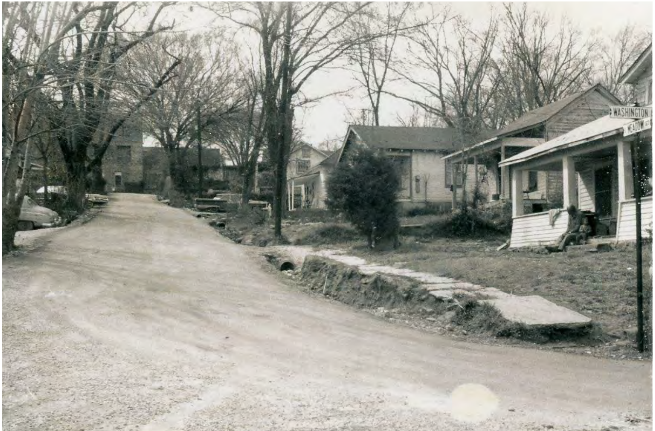
Figure 35. This ca. 1970 photograph of E. Meadow Street depicts unpaved streets, open drainage ditches, and hazardous sidewalks, all pointing to the City’s lack of investment in the infrastructure of southeast Fayetteville. These issues were among the chief complaints cited by residents in the 1968 Community Renewal Program document. Source: City of Fayetteville.
