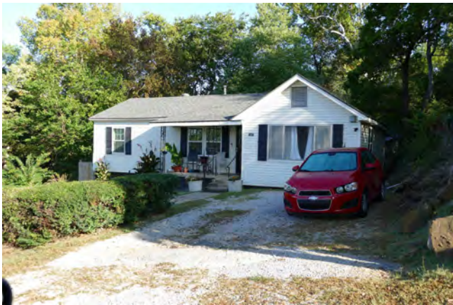
404 E. Center Street Approximate date of construction: 1951 (CAD) Form/Style: Gabled Ell/ "Bent House"
