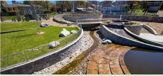
Close-up of a retention pond in Cook Park, where TPL oversaw the transformation of a green space in the Vine City neighborhood of Atlanta, Georgia, which had a history of severe flooding. © Astra Group and Jennifer Camacho
