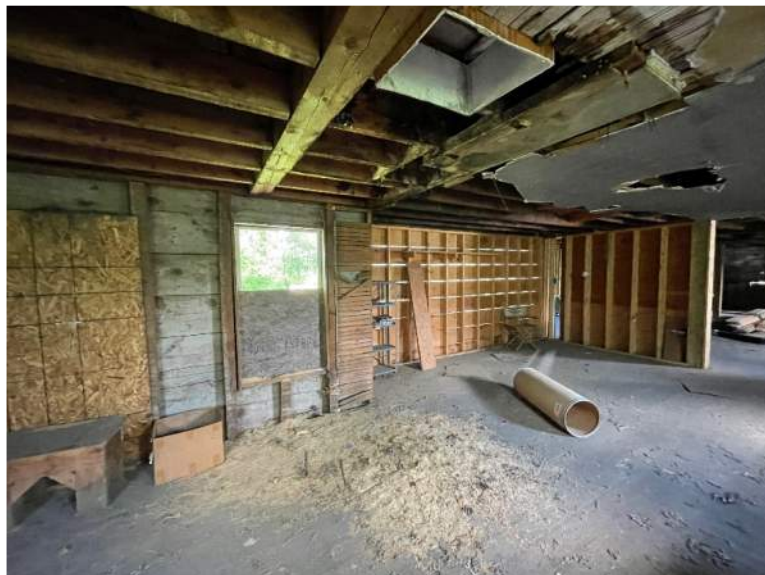
BACK HOUSE SECOND FLOOR FRAMING
