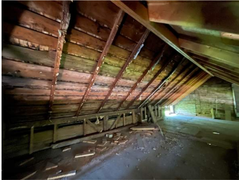
BACK HOUSE ROOF FRAMING
