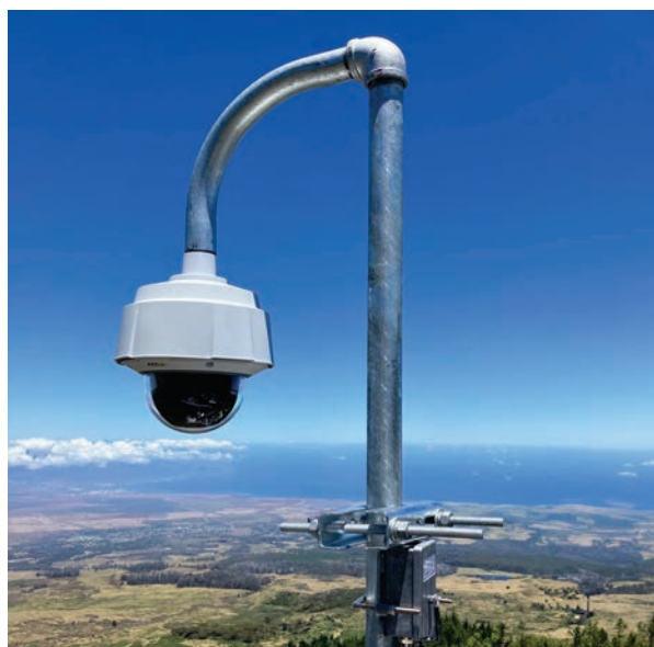
Figure 4-4. Sample Hawaiian Electric deployed AI-assisted video camera on Maui
