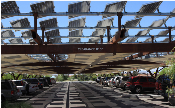
Solar panels above a parking lot provide shade and generate energy. Image source: Flickr user stuartwildlife
