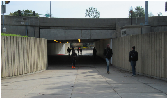
College Avenue/Main Street pedestrian underpass.
