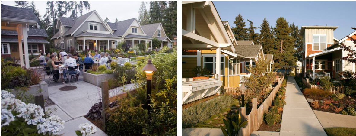
Cottage Housing Developments in Kirkland, Washington
