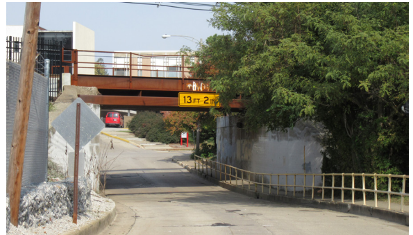
Union Pacific railroad bridge crossing School Street.
