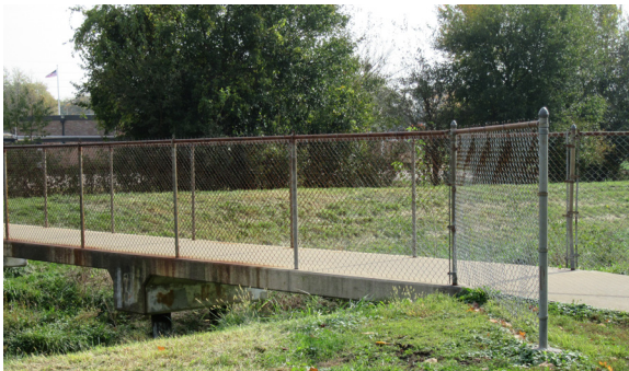
Pedestrian bridge connecting Oakdale Avenue to Oakdale Elementary School.
