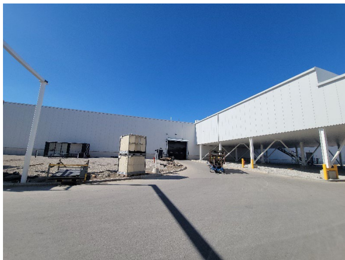
East Side of Main Plant
