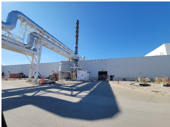
East Side of Main Plant
