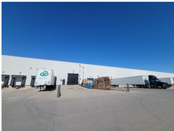
South Side of Main Plant
