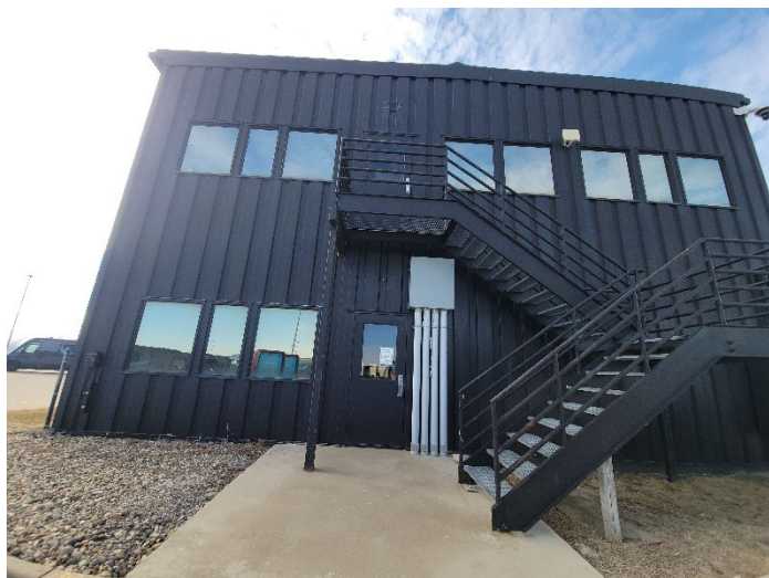
Decommissioned Outbound Logistics Building
