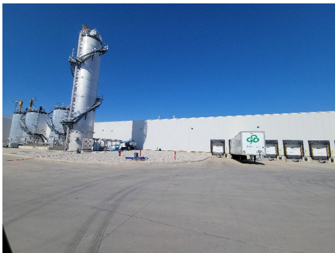
South Side of Main Plant
