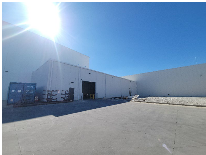
East And North Side of Main Plant
