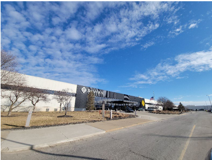
West Side of Main Plant – Main Entrance
