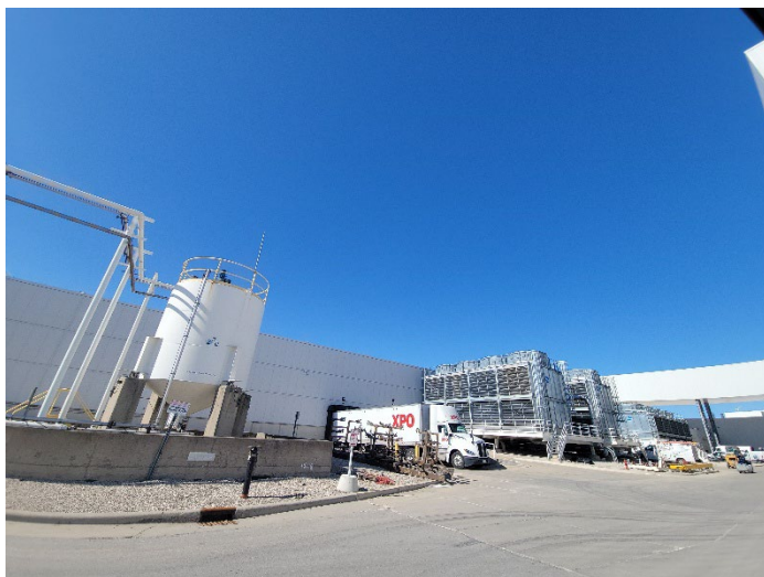
East Side of Main Plant
