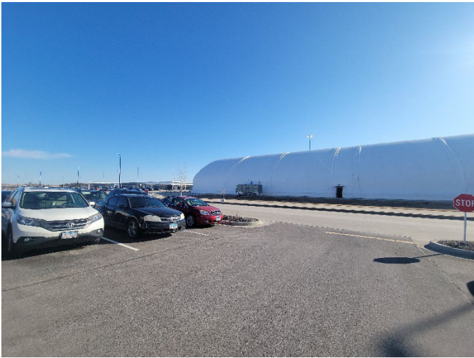
West Side of Main Plant
