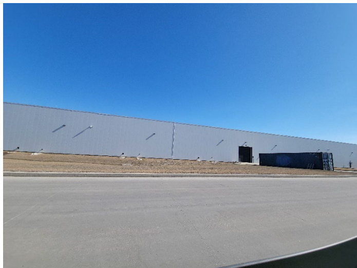
West Side of Main Plant
