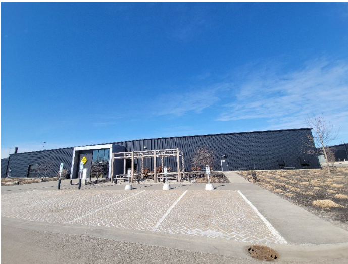
North Battery Building
