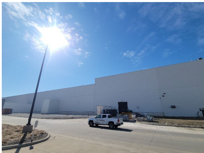
North Side of Main Plant
