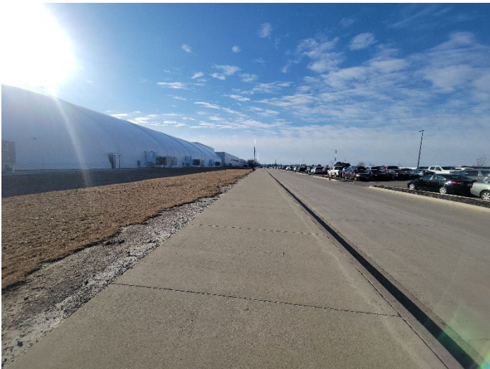
West Side of Main Plant
