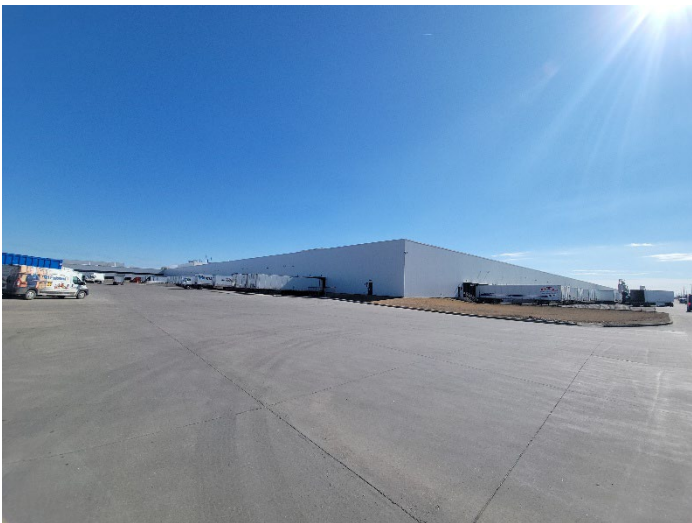
North and West Side of Main Plant
