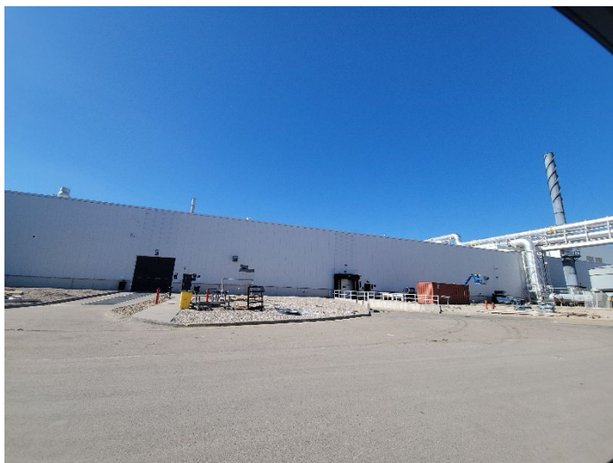
East Side of Main Plant
