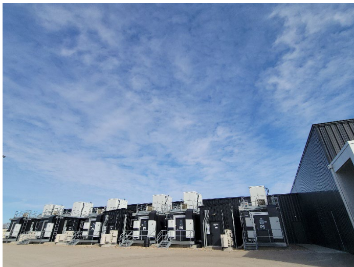
Exterior of North Battery Building Modular Units
