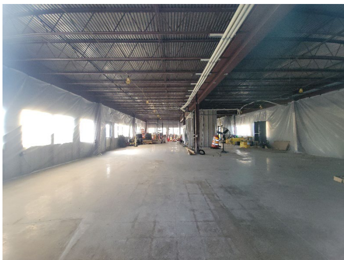
Decommissioned Outbound Logistics Building Interior
