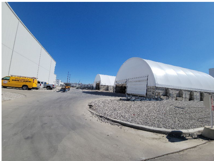
East Side of Plant
