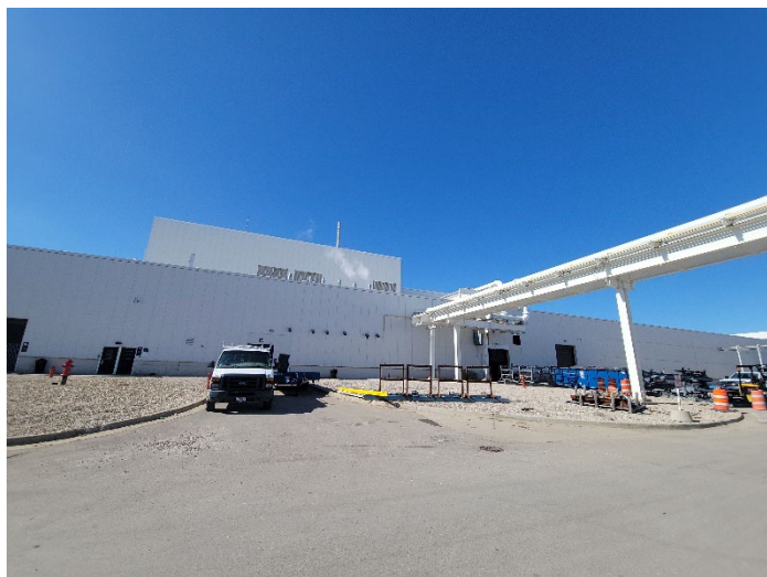
East Side of Main Plant
