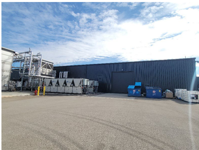
West Side of Battery Building
