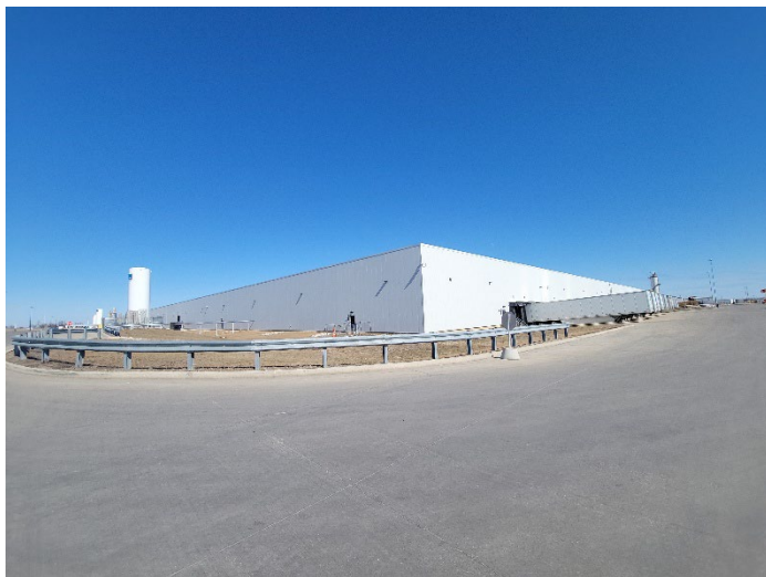
West and South Side of Main Plant
