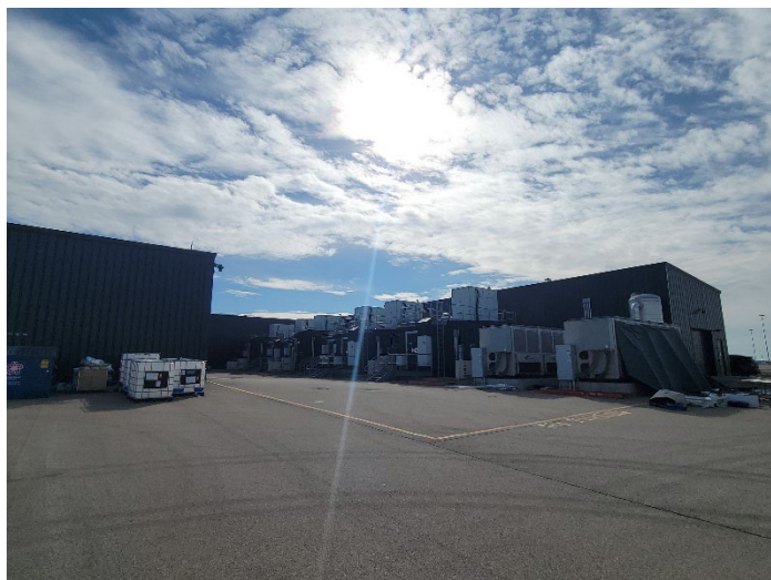
Exterior of North Battery Building Modular Units
