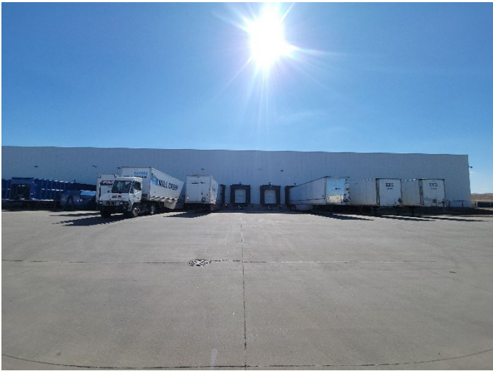
North Side of Main Plant
