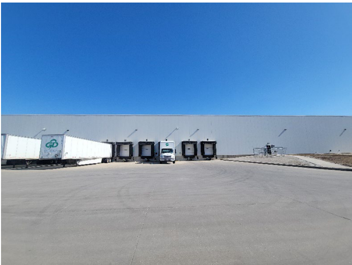
West Side of Main Plant
