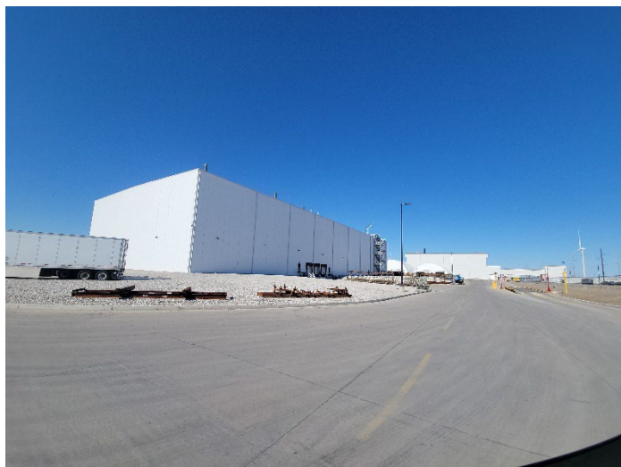
South and East Side of Main Plant
