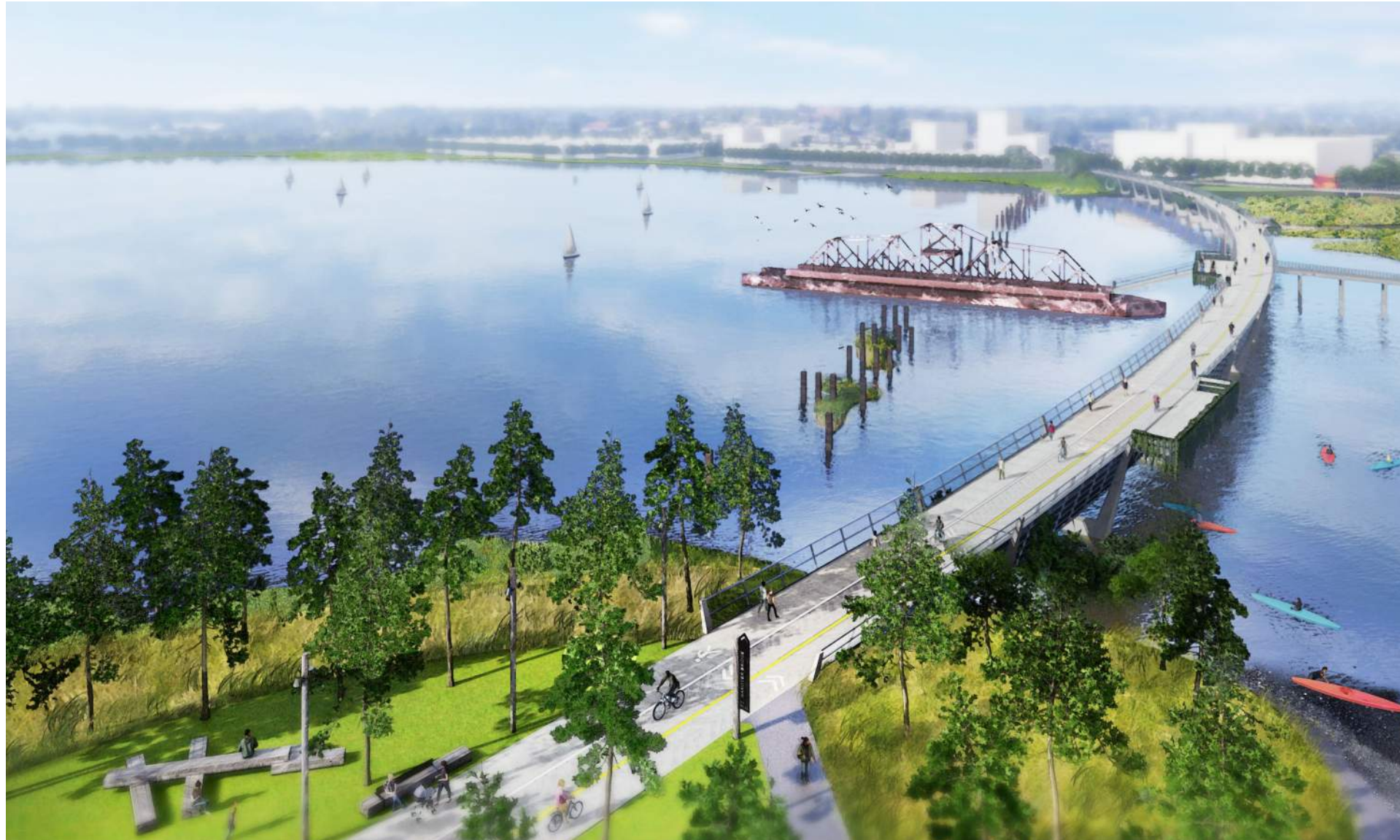
East-West Bridge connecting Port Covington to Westport looking west
