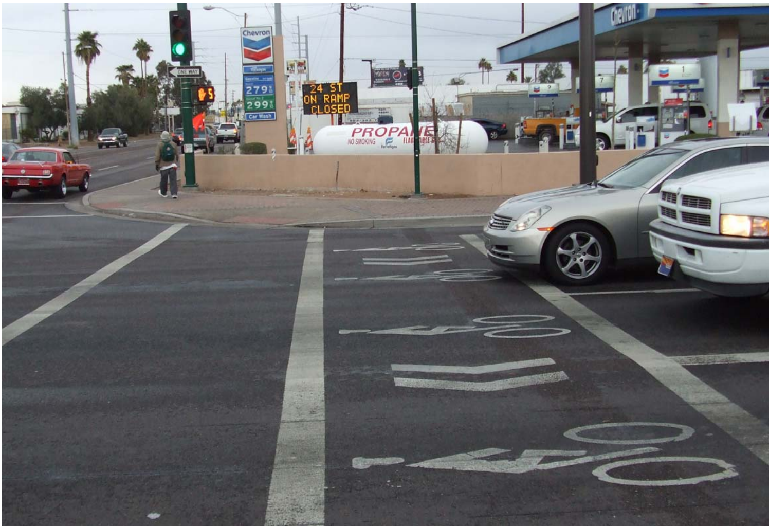
Figure 97: 24 th Street and Washington Street – Bike-Crosswalk
