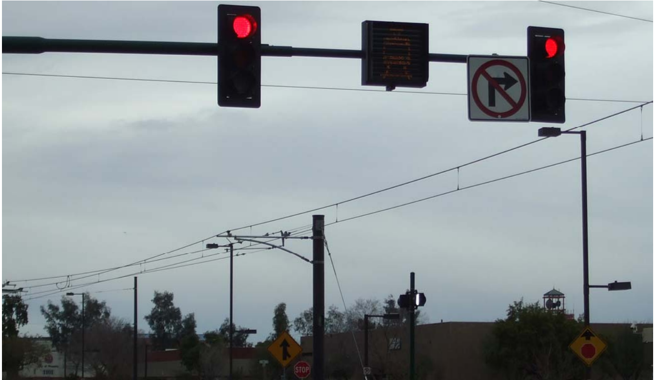
Figure 38: Crossover on Jefferson Street, East of 9 th Street – Existing Traffic Control
