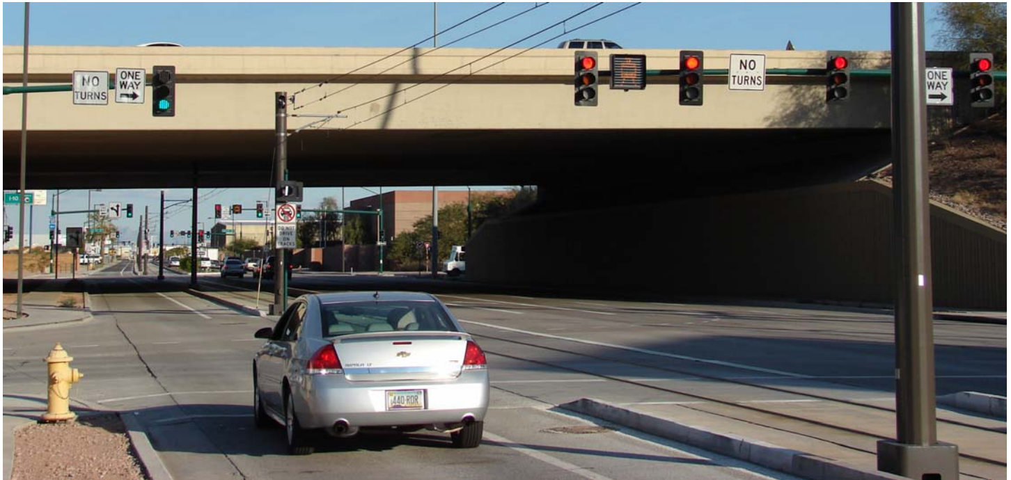
Figure 8: I-10 / Jefferson West Signal – LRT Go, Mainline Red, Frontage Green
