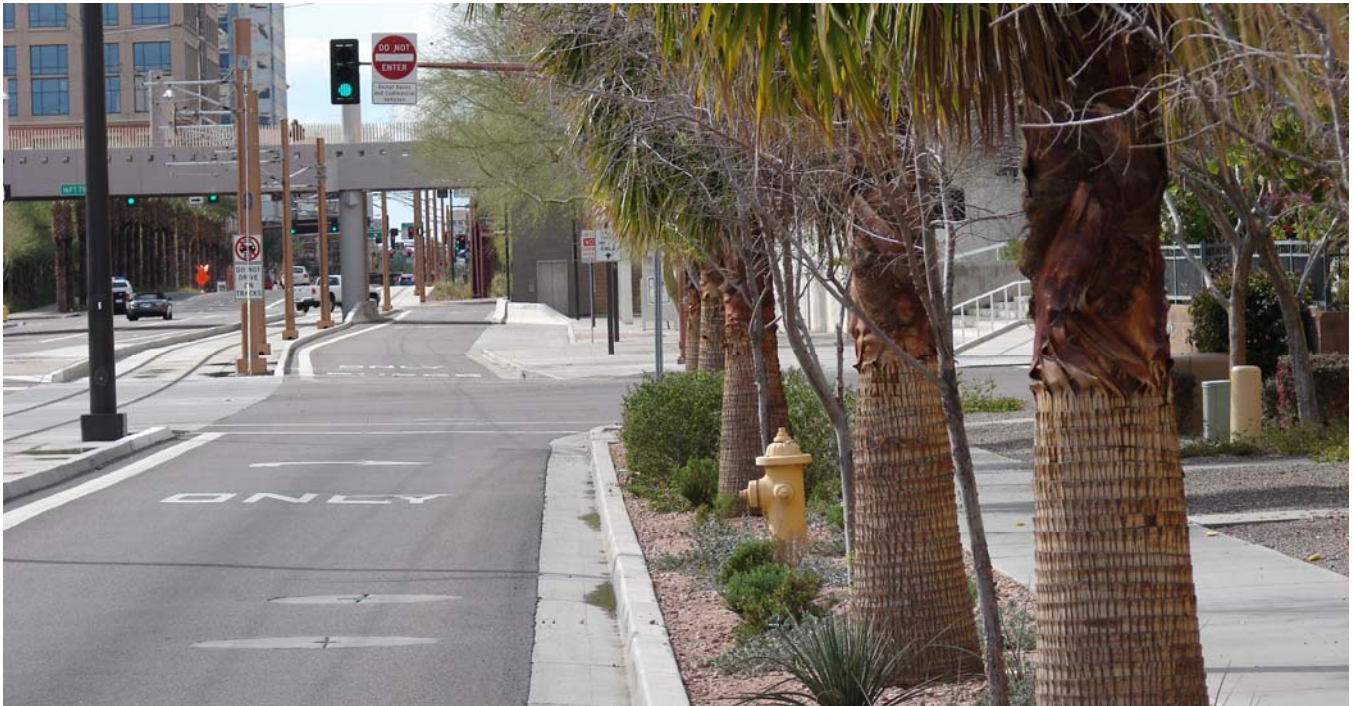
Figure 5: 700 East Washington Street – Right-side Frontage Road Turn-lane Approach
