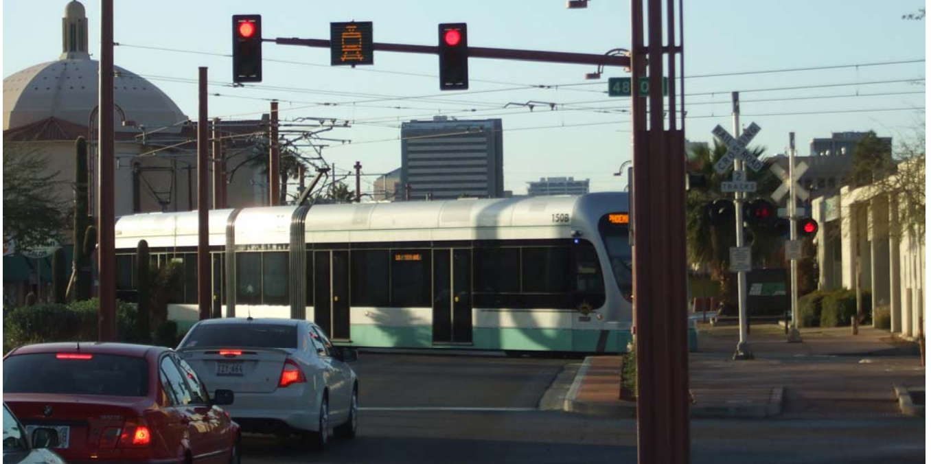
Figure 47: Central Avenue, South of Camelback Road – Existing Traffic Control
