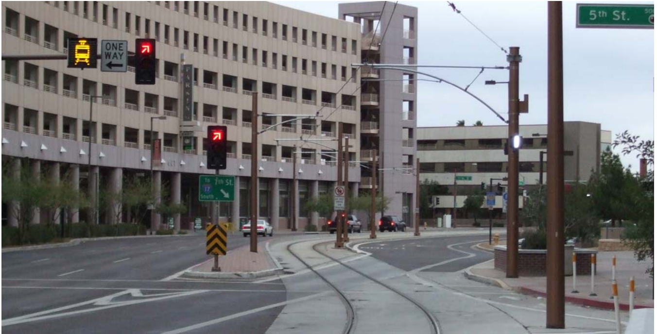
Figure 45: Crossover on Jefferson Street, East of 5 th Street – Existing Traffic Control
