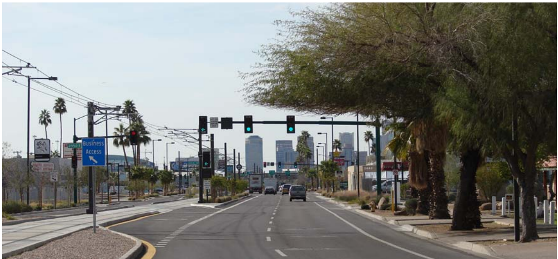
Figure 1: 2550 East Washington Street – Westbound Approach – Distant
