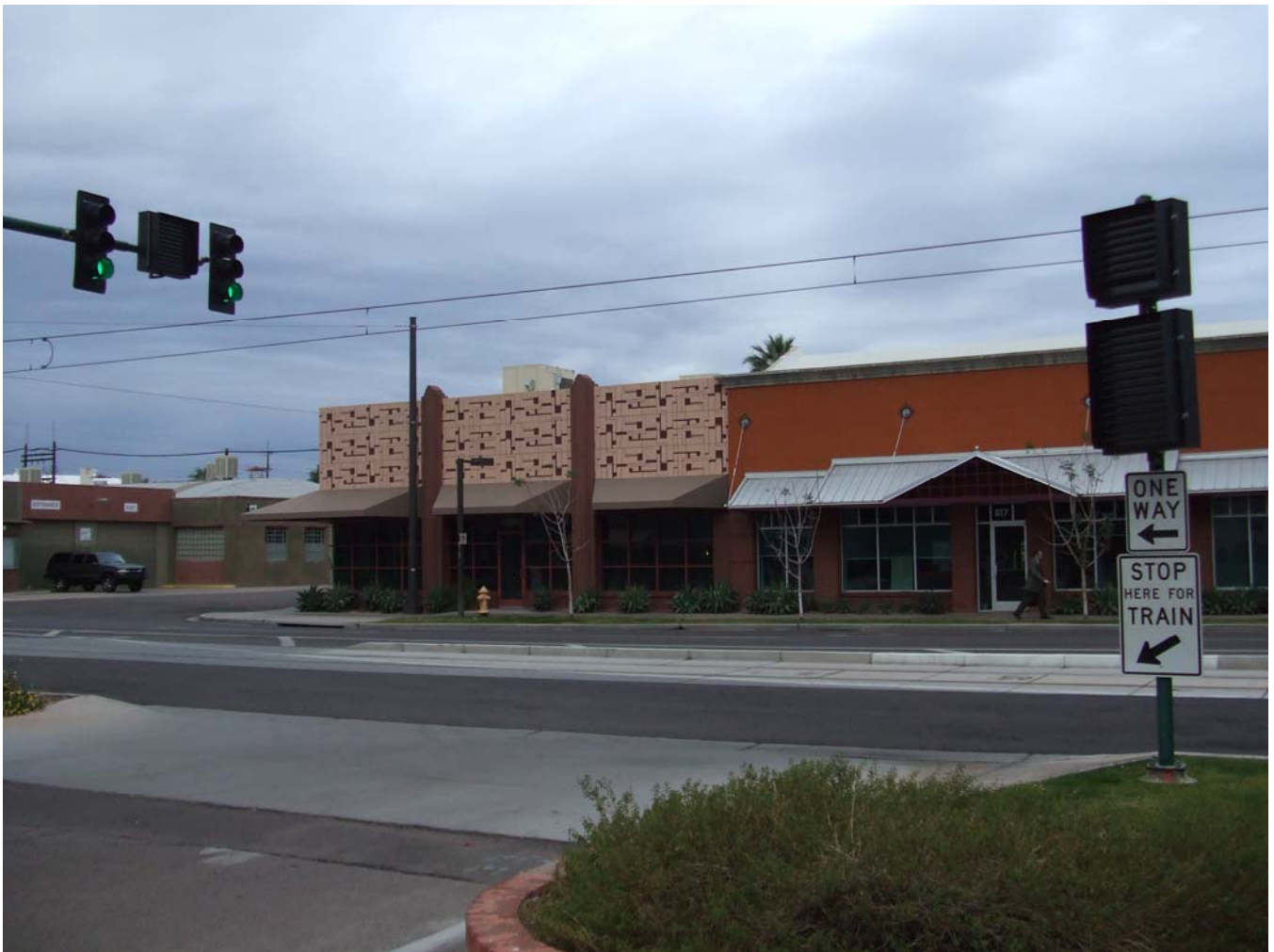
Figure 86: Central Avenue, North of McKinley Street – Access
