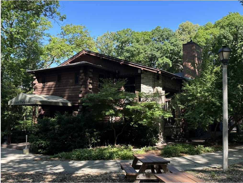
Photo 1: Main (south) lodge entrance
