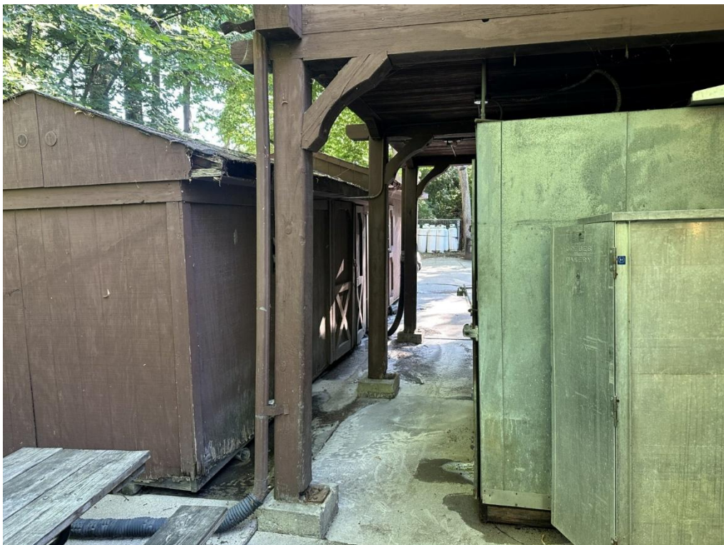
Photo 4: Three exterior wood columns supporting north side of caretaker's apartment
