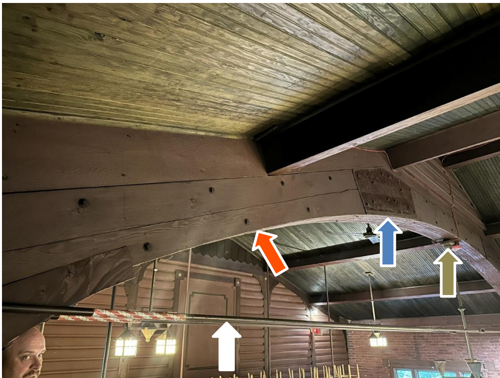
Photo 6: Wood roof girder. Orange arrow indicates end segment (sim on opposite end of truss). The green arrow indicates the center segment. The blue arrow indicates the gusset plate connecting the segments. White arrow indicates steel rods.
