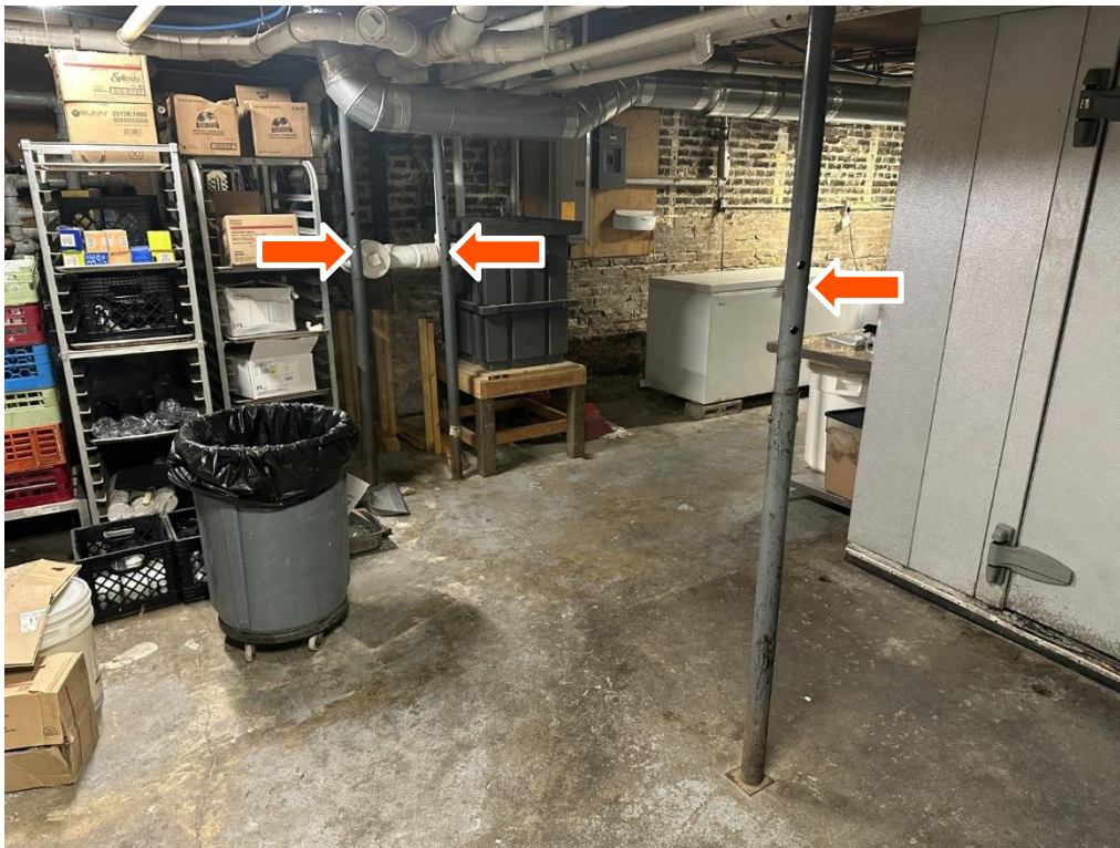
Photo 9: Pole shores supporting ground level floor framing
