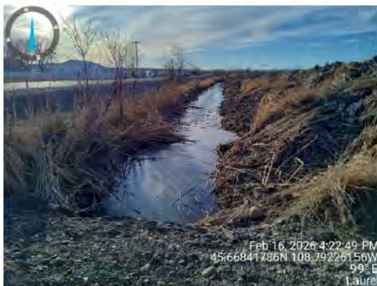
BED-AND-BANK-1, DREDGED SECTION
