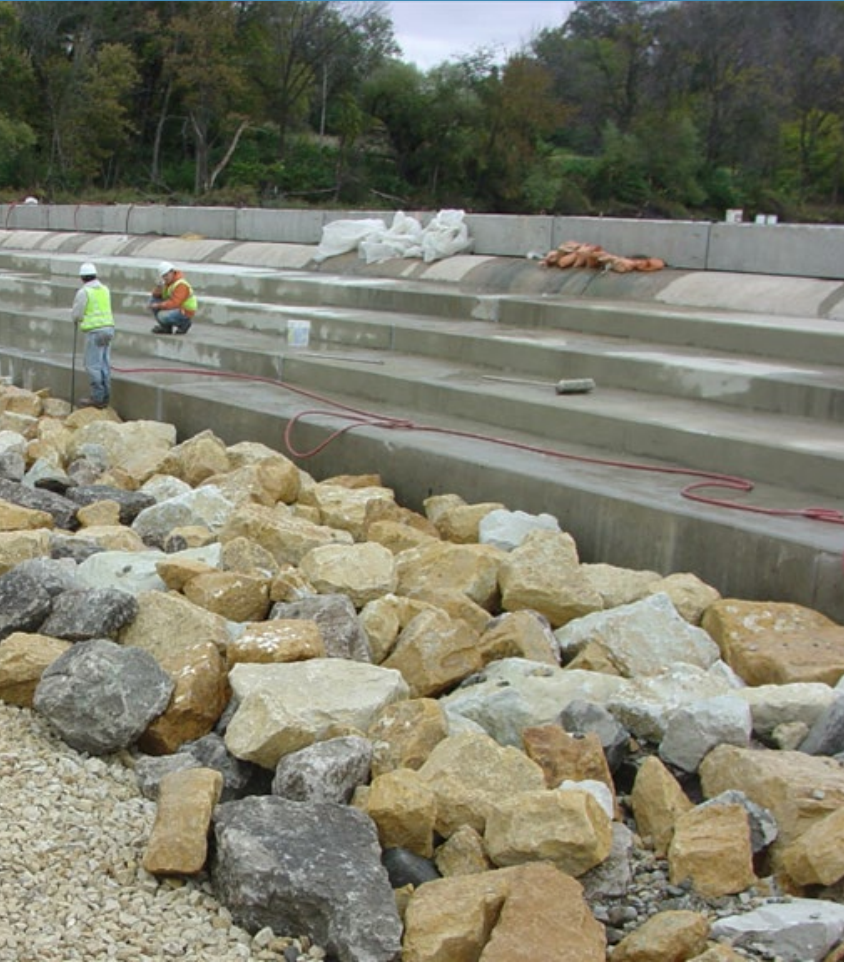
Stepped Spillway Yorkville, IL
