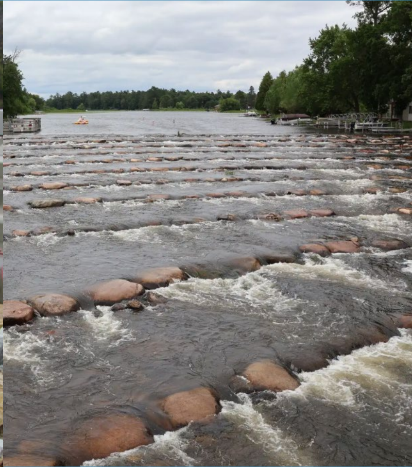
Rock Ramp Pine River, MN
